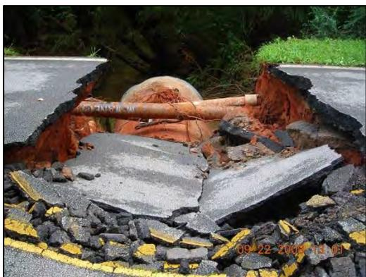
**Damaged Water Pipes on Brown Lee Road in Gwinnett County, GA during the September 2009 Flood.**
